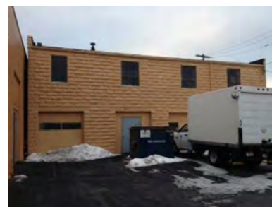
Old garage exterior.
