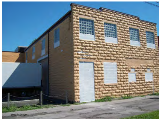
New glass block windows primed for final coat of paint.
