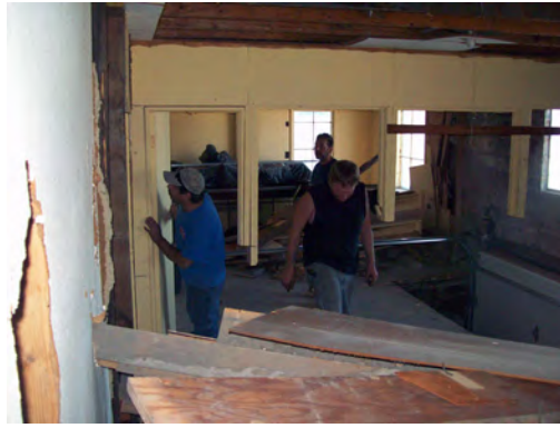
Second story demolition.
