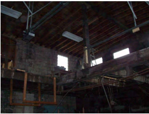
Demolition progress and new lighting.
