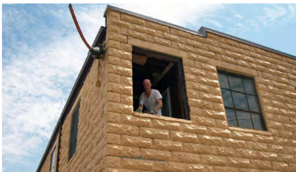
Second story window replacement.
