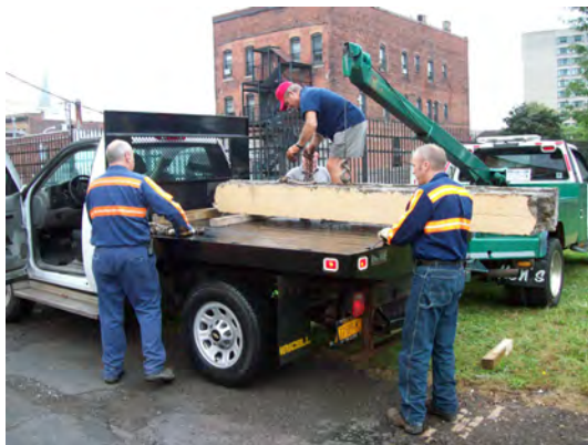
Removal of old concrete lintel.
