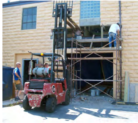
Masonry work on garage door.
